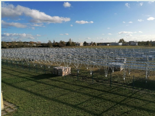
Figure 8: Our solar park is being built. Commissioning at the beginning of 2025.
